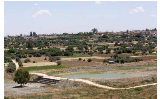
Gabion weir with recharge pond near Orounta village in the lower reach of the river. Photo Gerald Dörflinger; date: May 2013
