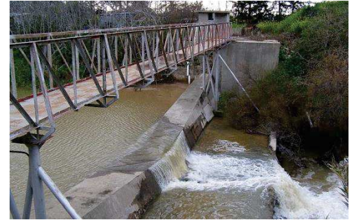
Flow gauging station on Ezousa River near Akhelia. Photo: Gerald Dörflinger; date: February 2009
